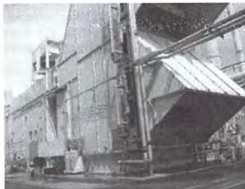
Figure 1A – Kingsburg Inlet Duct Configuration
