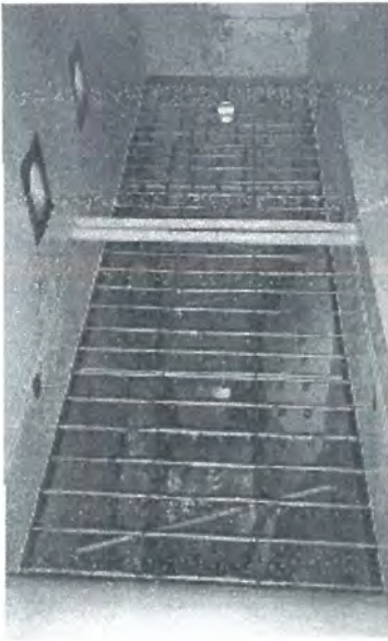
Figure 2: Nozzles Arrays mounted in the duct.
