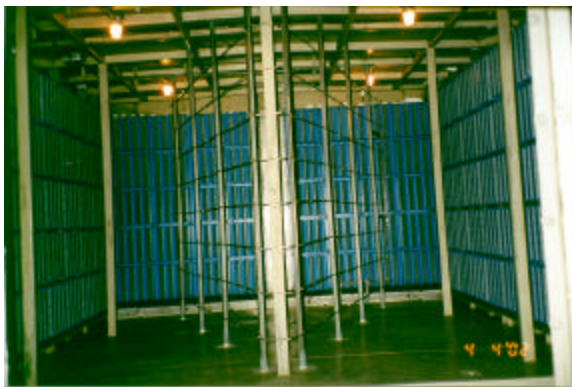
Figure 3: Nozzle layout in the inlet duct.
