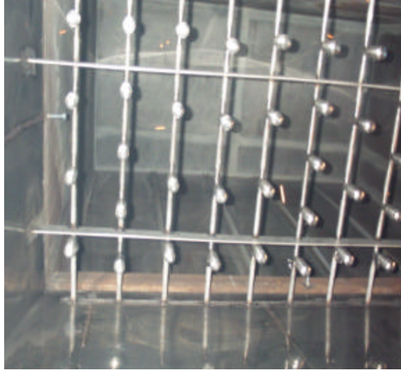
Figure 6: Installation of spray nozzle rack in the inlet duct.
