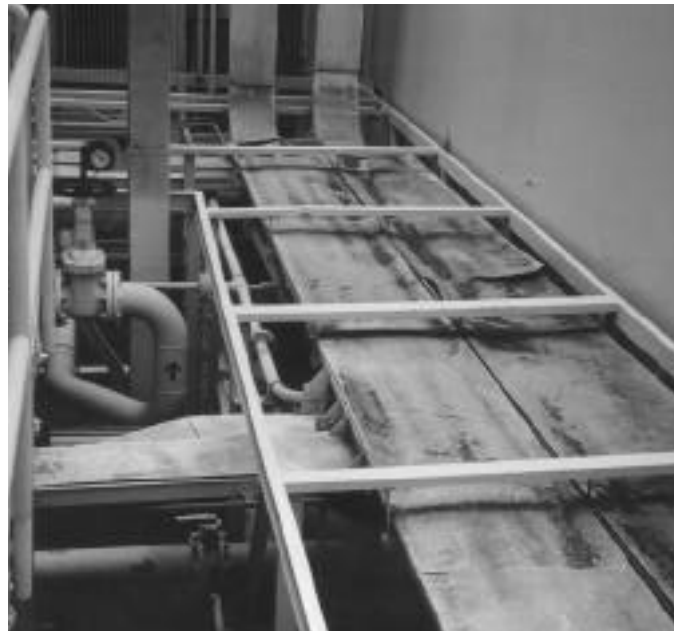
Fig.8: Space available for pump skid.
